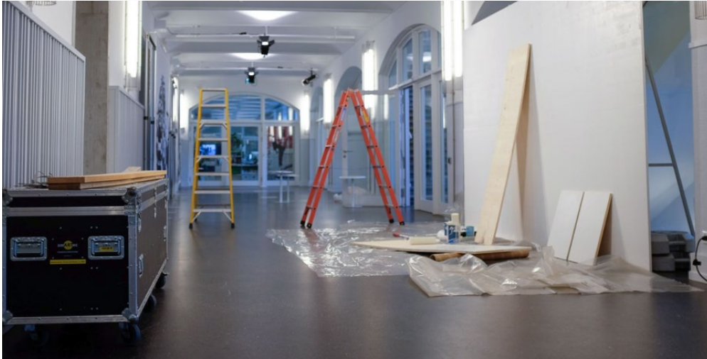
Figure 6: Remodelling work in the main building of the Kaserne
